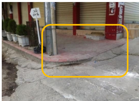
Fig.16: Lack of standard curb ramp into the sidewalks of the study area (Source: Researcher)
