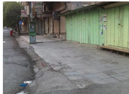
Fig.13: Various materials in different colors, textures and thickness were used in the finishing of the walkways. (Source: Researcher)
