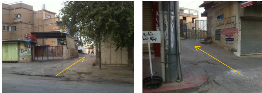
Fig.17: The drive way crossing has not been considered into the sidewalks of the study area. (Source: Researcher)
